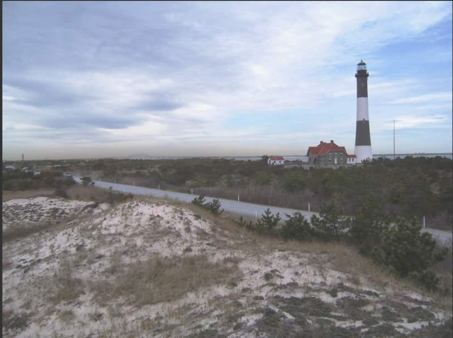
Fire Island – Aggregate Surfacing
